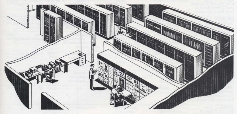
proved construction of a digital computer in 1946. A general-purpose computer could take care of not only flight simulation calculations, but a variety of other scientific and engineering applications. Whirlwind was completed in stages; the entire central machine was working in 1951.
